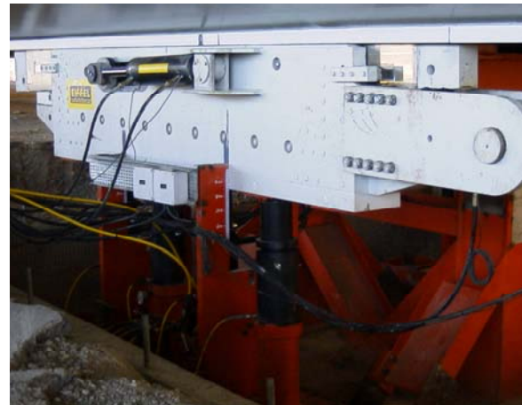
Fig. 1, 2: Installed launching device to forward the superstructure
