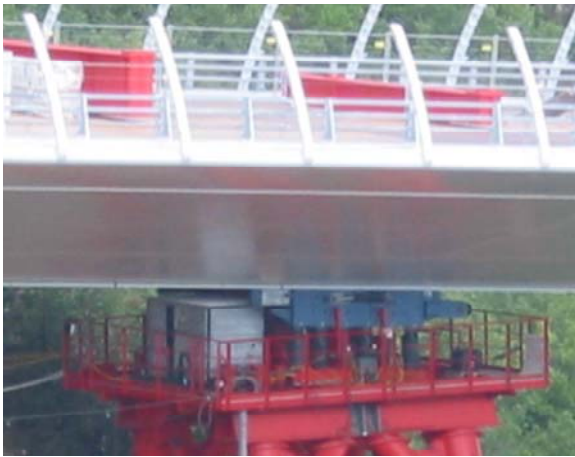
Fig. 1, 2: Installed launching device to forward the superstructure
